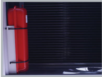
closed expansion tank
